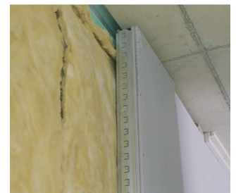
PARTY-WALL SYSTEM INSTALLATION
